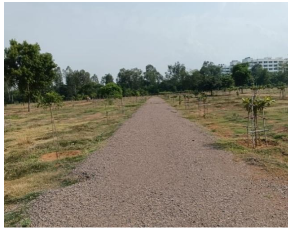
Providing wet mix road at new car parking area
