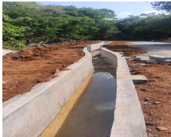
Construction of rain water channel
