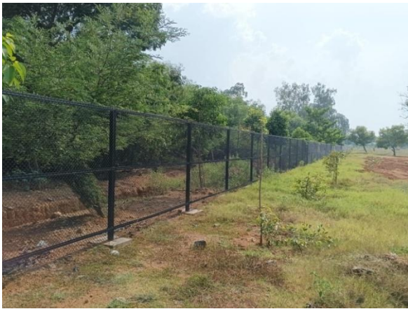
Erection of chain-link fencing between additional car park area and rescue centre
